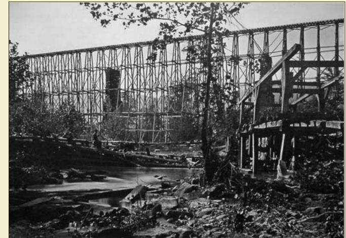
RUNNING WATER CREEK BRIDGE BUILT BY THE FEDERAL ARMY
